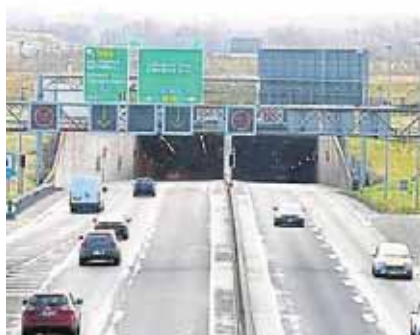
The closure will facilitate essential works on the Limerick Tunnel
