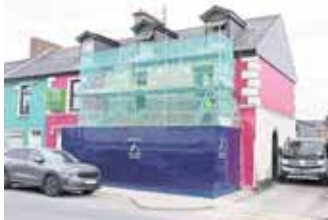
The former Sean Collins & Sons pub in Adare which was bought by the McManus family and is currently being refurbished PICTURE: ADRIAN BUTLER
